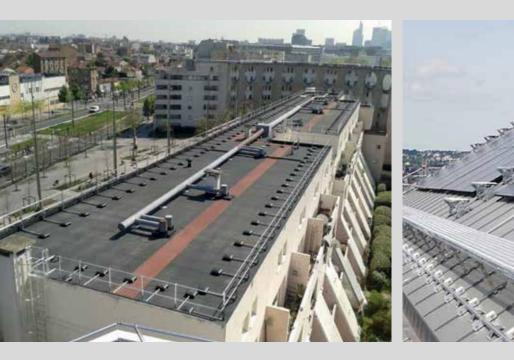
**GARDCO** safety rails can replace lifeline systems and safety posts. According to DIN 4426 guardrails should have priority to personal protective equipment (PPE) because they eliminate the fall hazard for all the workers on the roof simultaneously.
