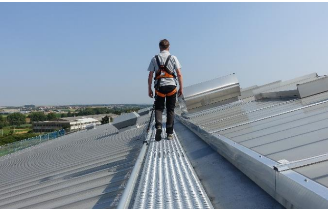
ROOFWALK SAFE Safety with fall arrest system e.g. for maintenance of SHEVS
